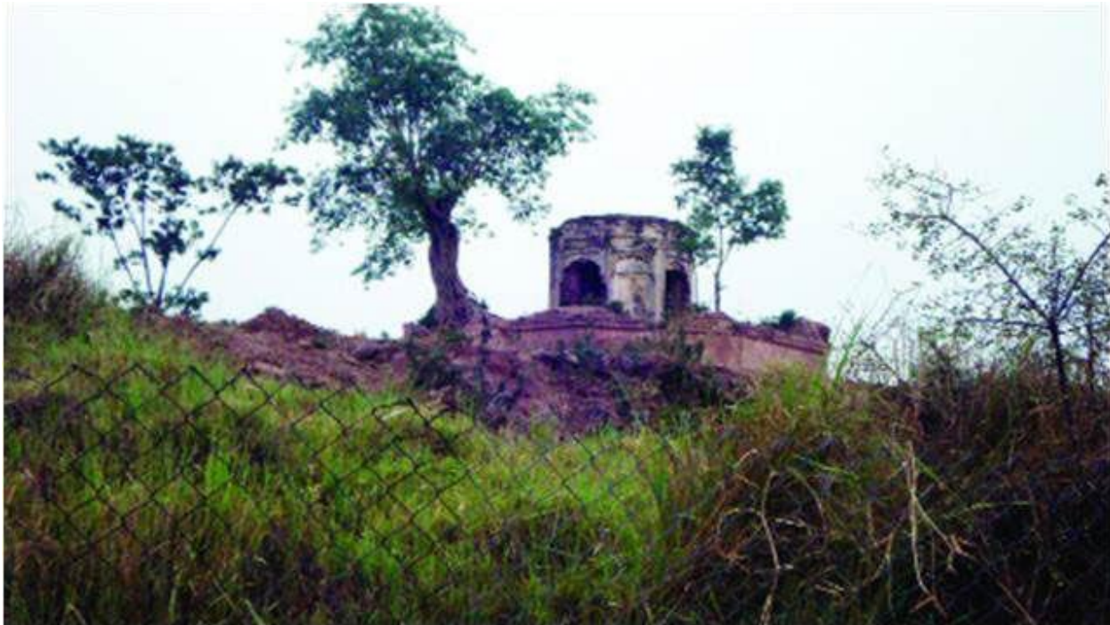
Fig.3. Ditrurbed complex of baradari need to be preserved ( By researcher)
