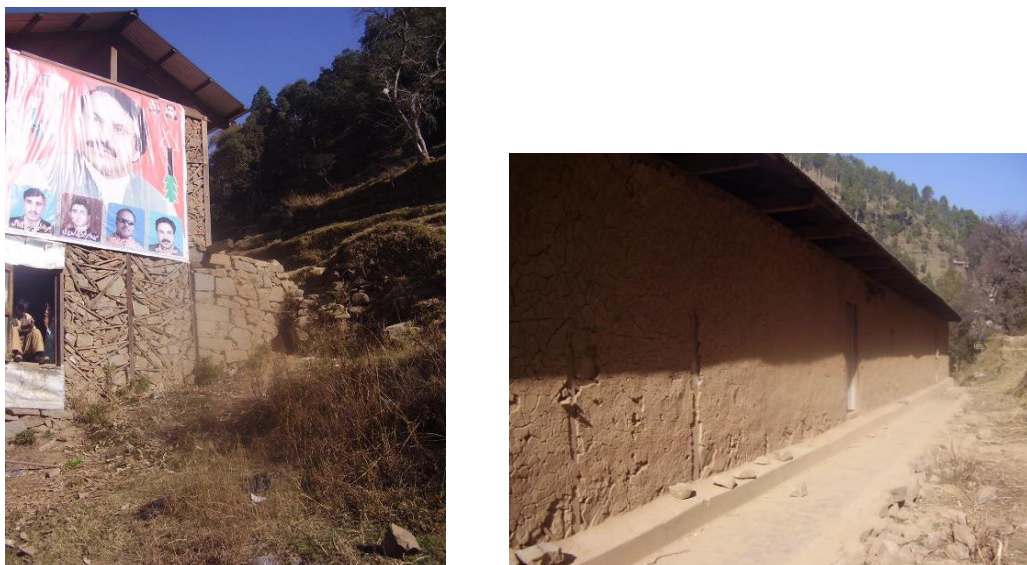
Figure 5: Pre-quake dhajji-built market in Bagh which survived the M 7.6 earthquake. Dhajji is not visible in right view as walls are covered with mud plaster on rear side of the building. Source: Author
