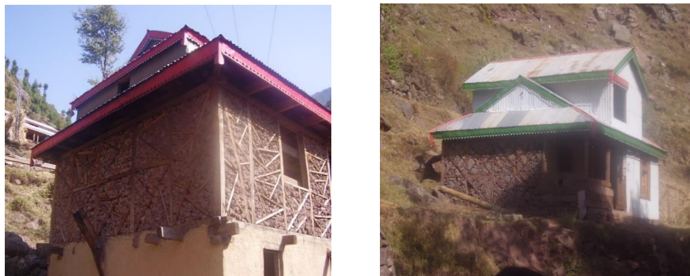
Figure 4: Typical two room houses in Dhajji dewari found near Muzaffarabad. Source: Author
