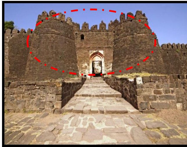
Figure 15: Daulatabad Fort near Hyderabad 1187 Red Circle indicating Arched Parapet.
