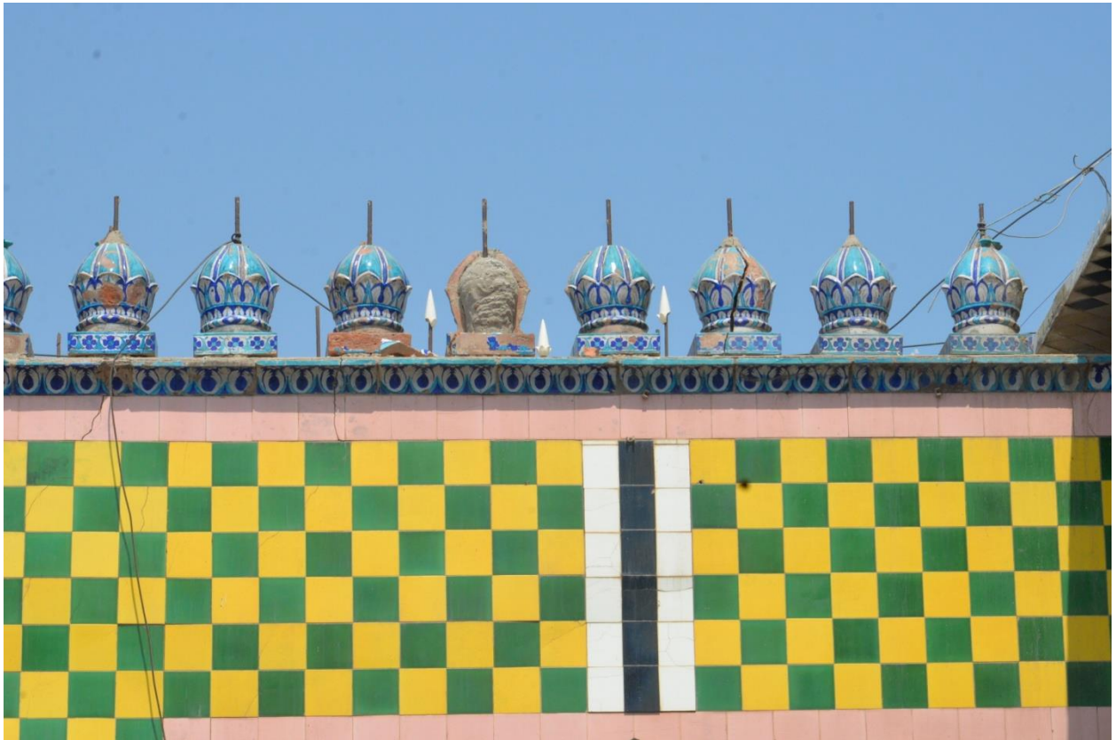
Figure 29 Green and yellow checked pattern on the façade
