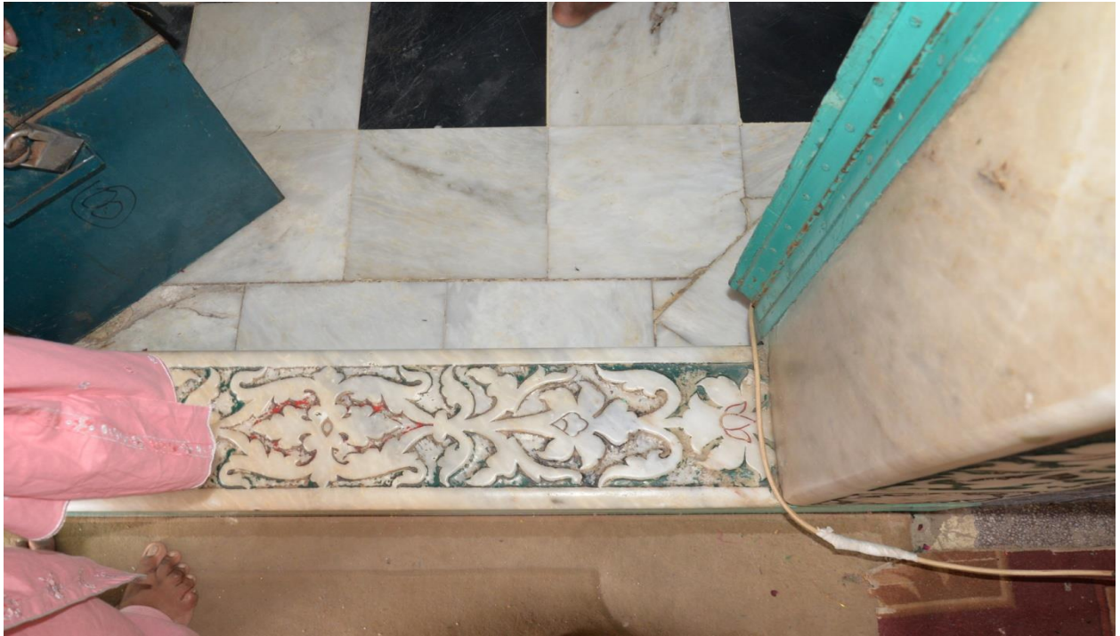
Figure 18 carved marble foot stone at the entrance door
