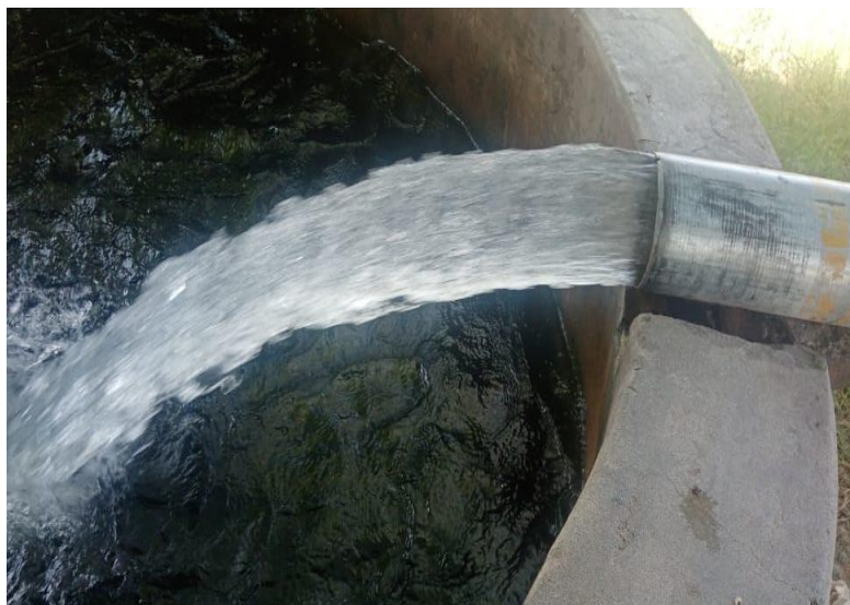
Fig 5: Discharge of water
