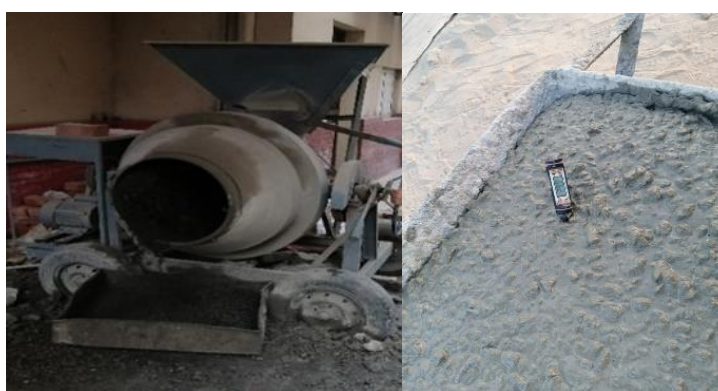
Fig. 2: Mixing of concrete
