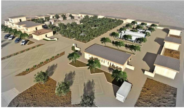
Figure 9. General view of the area.
