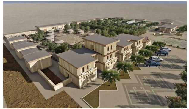
Figure 10. General view of the area.
