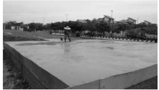
Fig. 4 - Preparation of concrete base based on the original size and height.
