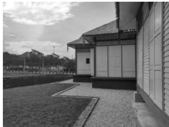
Fig. 7 - Pictures show the installation works of building elements and components of Teluk Memali Mosque including the fascia boards, mimbar treatment, balai lintang construction and landscaping work.
