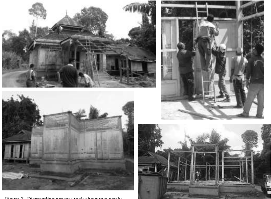
Figure 3- Dismantling process took about two weeks.
