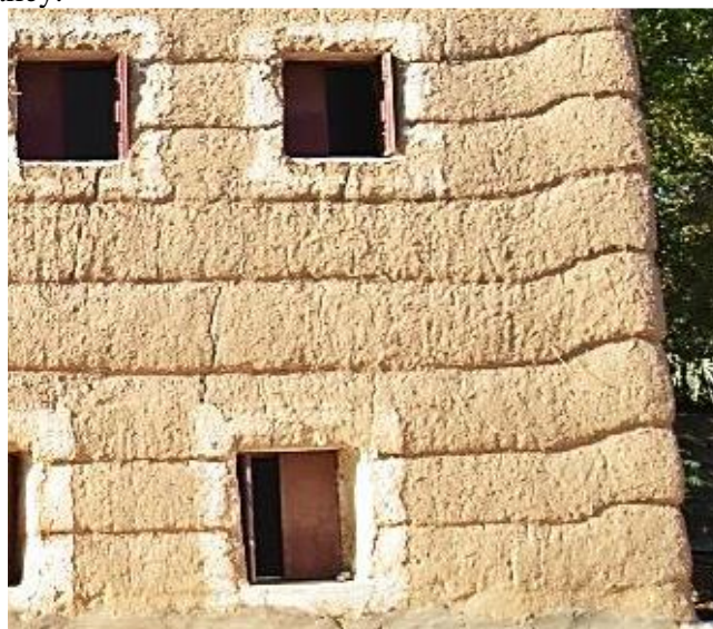
Figure. 4: The tradition of mud “cob” architecture in the Zakho valley
