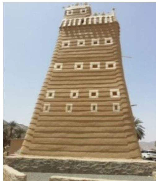
Figure. 2: Zakho (traditional earth building).
