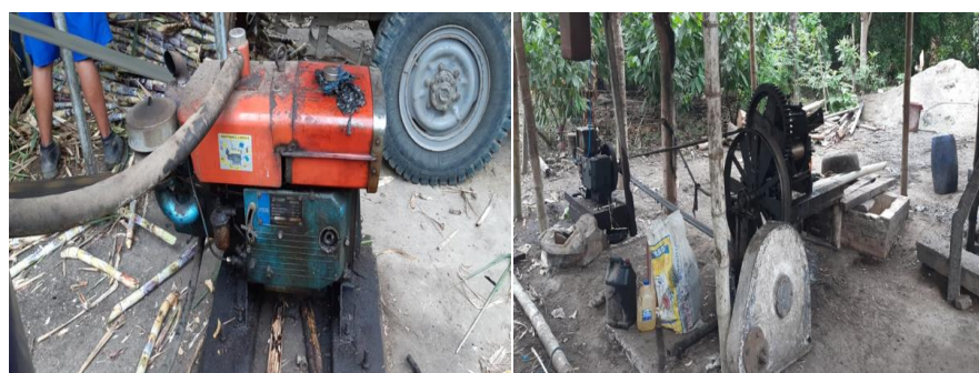
Figure 2 Diesel generators used in small industries
