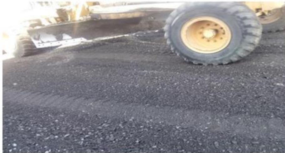
Figure 5.5: RAP Aggregate Base course / WMM Placement
