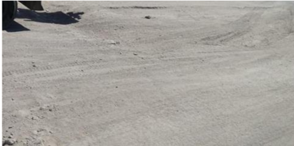
Figure 4.5: Distress Road section location before laying.
