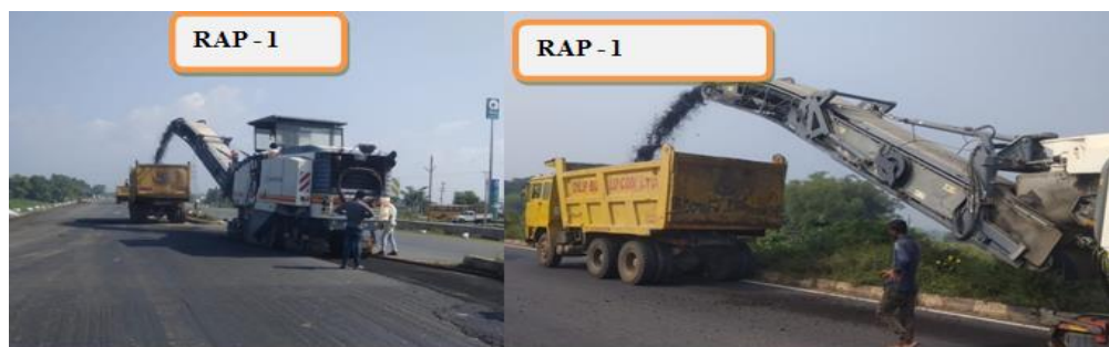
Figure 4.1: @ km. 119+000, Milling Area
