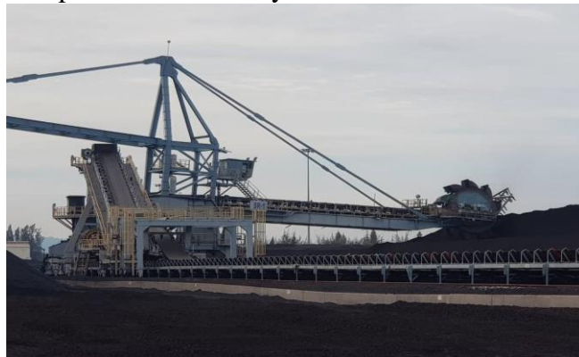
Figure II: Stacker at coal yard
