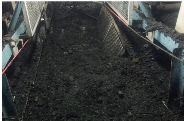
Figure III: Coal transport via coal conveyor line
