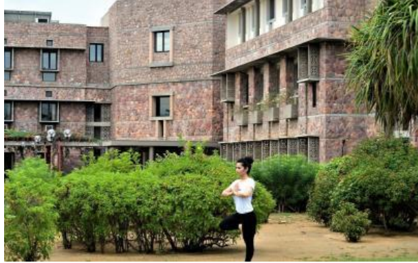
Fig. 20 Building clad with stone and solar panels on the rooftop (Source- A+D, Mar-Apr, 1993, May 2020)
