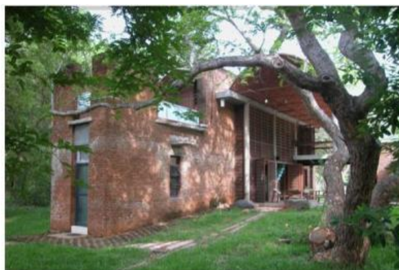
Fig. 9 External View of the Wall House
