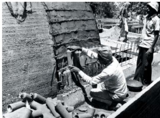
Fig. 4 Construction of Barrel Vault in Sangath (Source- https://architexturez.net/doc/az-cf-168122 , April 2020)
