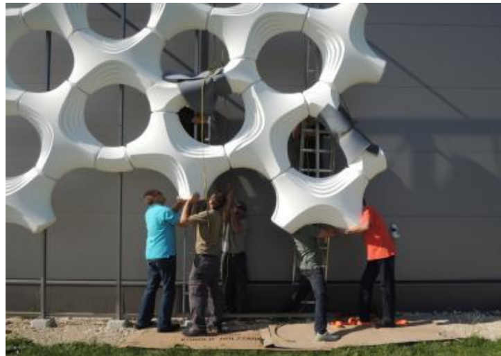
Fig .3. Installation of the prosolve tiles [13]
