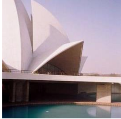
Fig 17. View of the pool [23]
