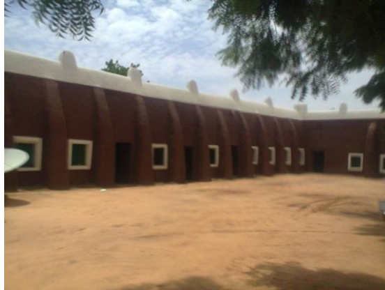
Plate II: Side view from the courtyard of the Katsina collage showing elements of Islamic and Hausa traditional architectural style; author's fieldwork
