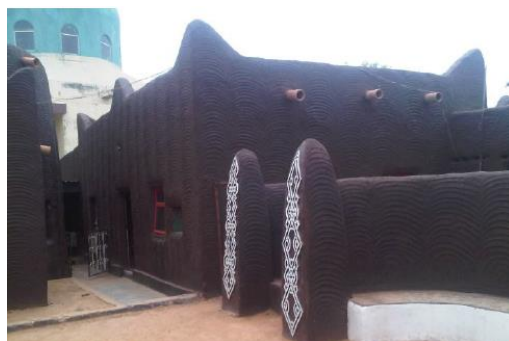
Plate IV: Side view of the gallery from the courtyard showing different traditional architectural elements like the pinnacles, motifs, sprouts, mud walls and others; authors fieldwork
