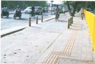
Photo 6 Levelled Crossing Over Cycle Track, BRT Corridor, New Delhi
