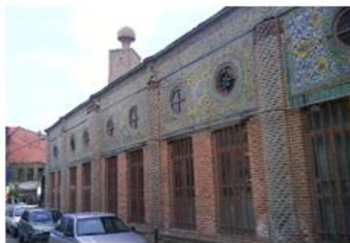
Figure 3: Sardar Mosque (openings)
