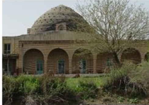
Figure 1: Homamian Mosque (openings)
