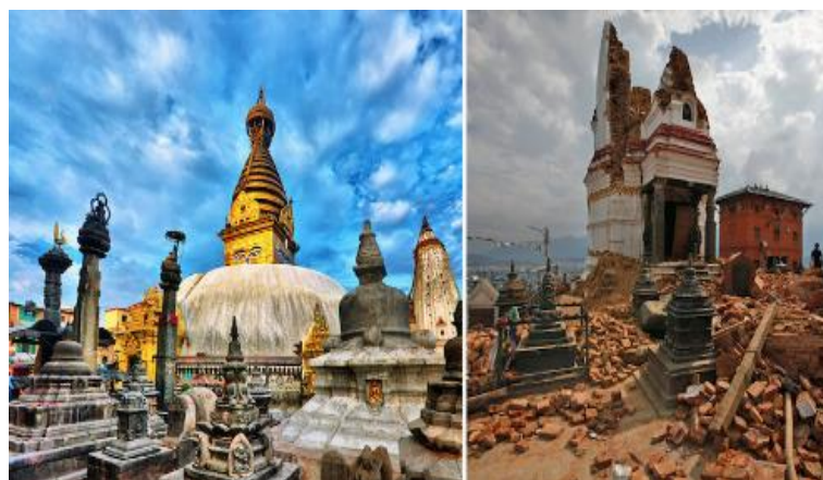
Fig. 3: Swamp Temple before (left) and after (right) of the 2015 Nepal earthquake (internet photo)
