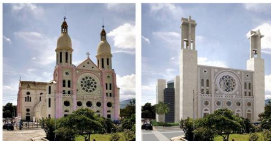
Fig. 12: Our Lady's Cathedral before the 2010 Haiti Earthquake (left) and after the Reconstruction (right) (Internet photo)
