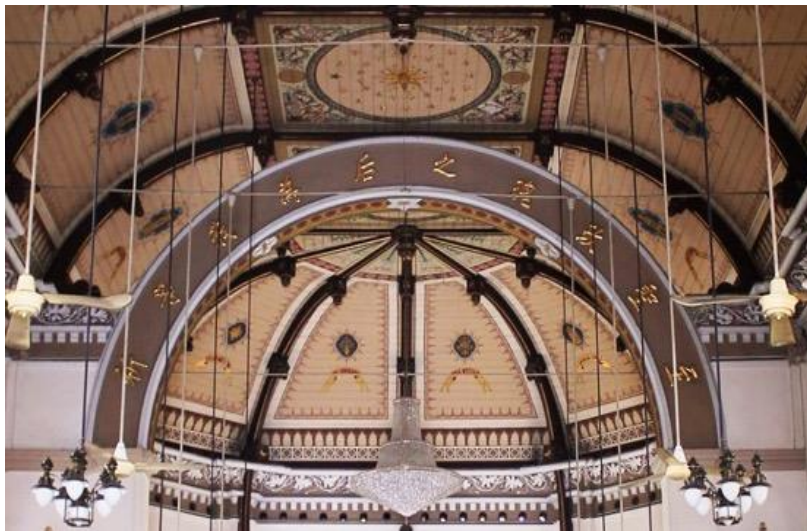
Figure 7: Chinese Inscription On The Ceiling Vault
