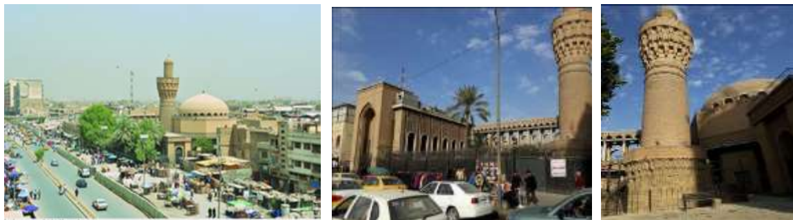
Pictures showing the minaret's inclination towards the east in a clear way, closing the mosque and announcing it with an announcement indicating the presence of maintenance in the mosque and the other showing the urban scene and the presence of the spinning market and the mosque in the early morning hours. Source Researcher
