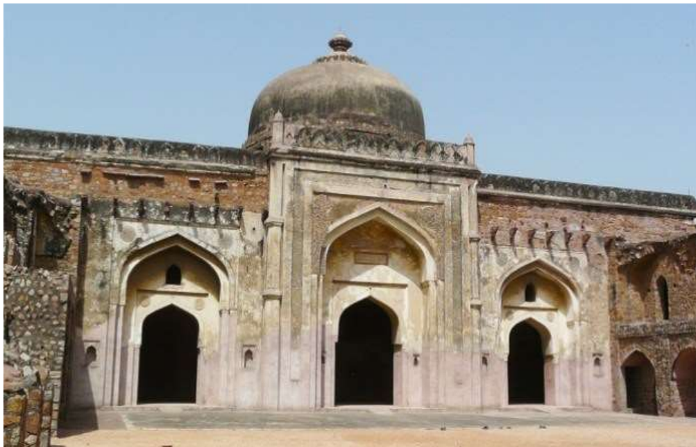
KharulManazilmasjid build by MahamAnga 1561,New Delhi
