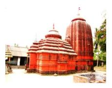
jagamohana of the temple was built during the Somavamsi time frame. The jagamohana is saptaratha in arrangement. The pabhaga of the bada measures 2 feet 4 creeps in stature. The tala jangha of the bada is totally plain. The bandhana of the bada comprises of two even moldings, which are joined by vertical band at the focal point of each paga. The baranda of the bada contains 9 flat moldings, which are joined by the upward band at the focal point of each paga on all sides.
