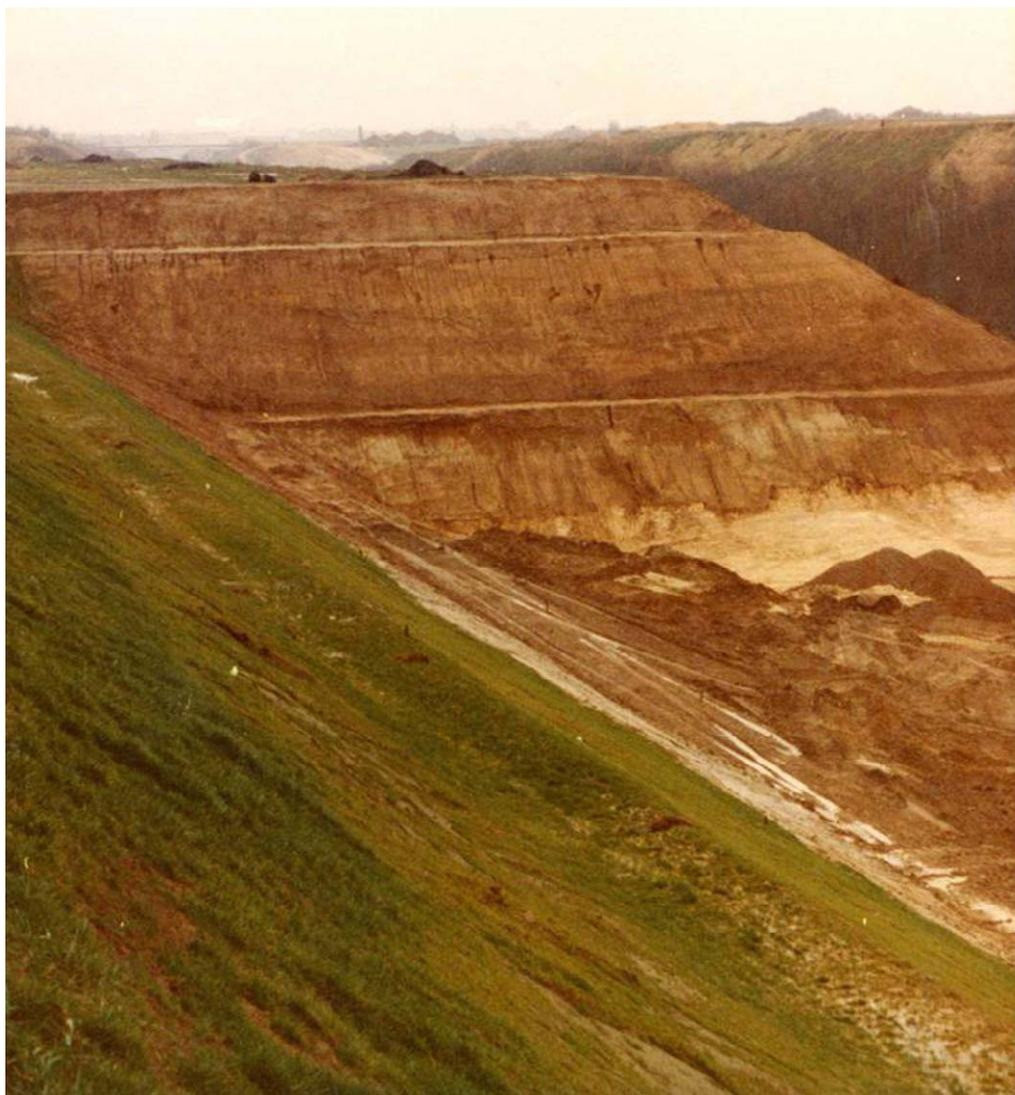
Figure 5. Widening of the Albert Canal at Kesselt in 1983, showing a succession of limestone (bottom), Tertiary sand, Maas gravel and loess, with a succession of five different interglacial soils, on top. Photograph by the author.
